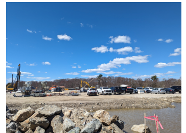
Above and below left: Current state of construction at 200 Quannapowitt Parkway
